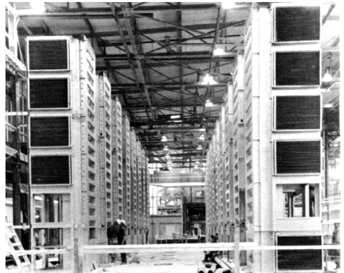
Figure 1: Construction of an Airborne Dryer
